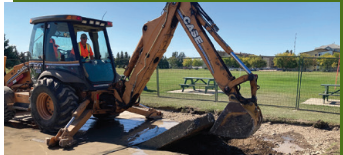
Splash park demolition.
