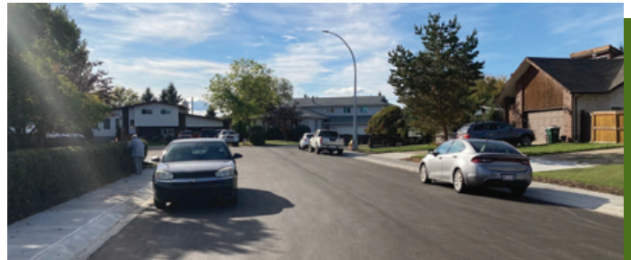
Residential Road Rehabilitation Project.
