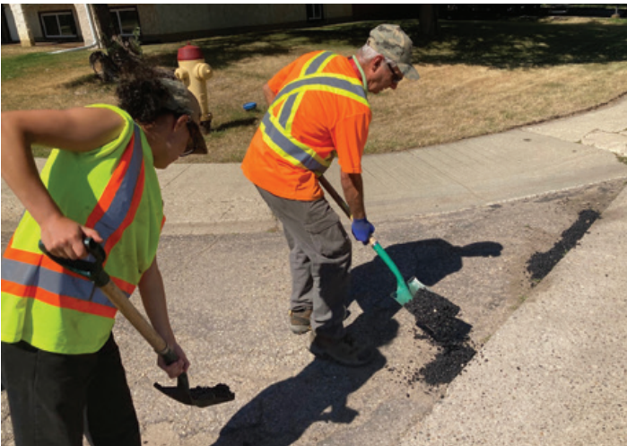
Pothole repair work.
