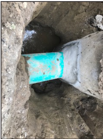
Storm line / CB Repair
