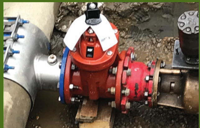
Industrial tie-on to waterline
