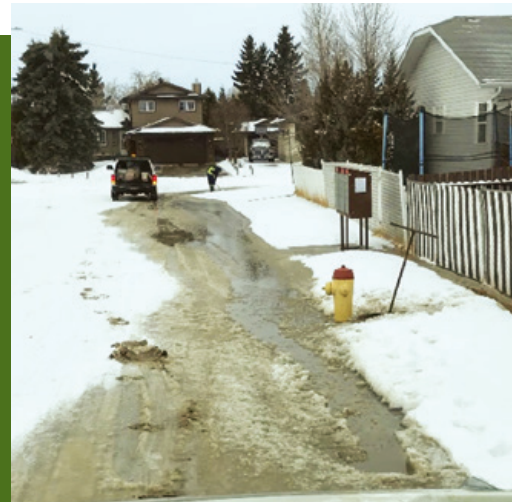
Hydrant leak
