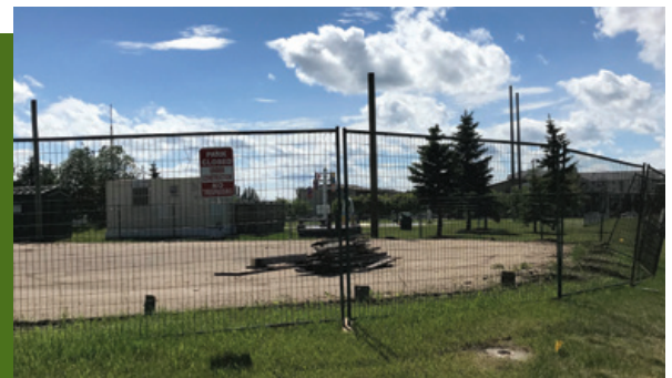
Outdoor rink demolition.
