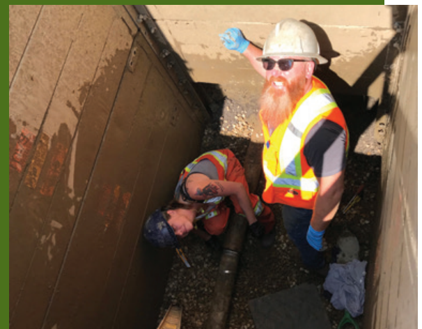
Road Rehabilitation Project hydrant repair.
