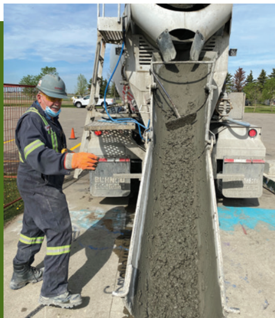
Concrete work at Bob Foster Extreme Skate Park.
